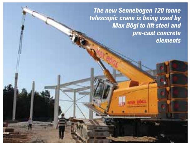
The new Sennebogen 120 tonne telescopic crane is being used by Max Bögl to lift steel and pre-cast concrete elements
